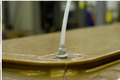
4- Then, the two-step Offshore Installation Process is carried out: A qualified Surface Preparation is performed prior to the Vacuum-Assisted Injection of the structural polymer (epoxy resin).
